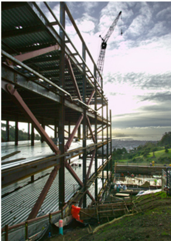
A Construction Project at LBNL
